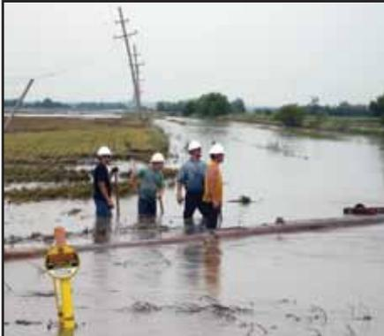
Ellsworth linemen work in flood waters, replacing power poles after receiving seven inches of rain from a spring storm.
